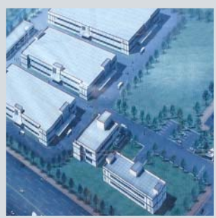
Wuxi Plant (China)
